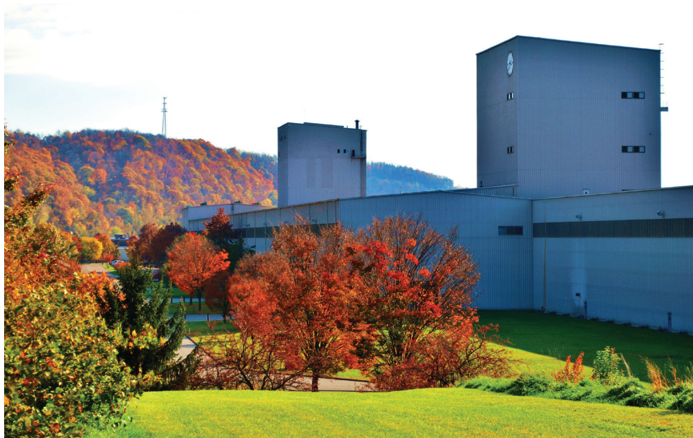
Wheeling-Nippon's facility in Follansbee, West Virginia.
